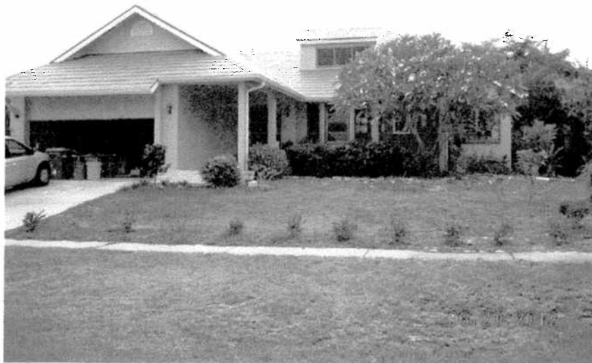
FRONT VIEW (SOUTHWEST) June 20, 2012
