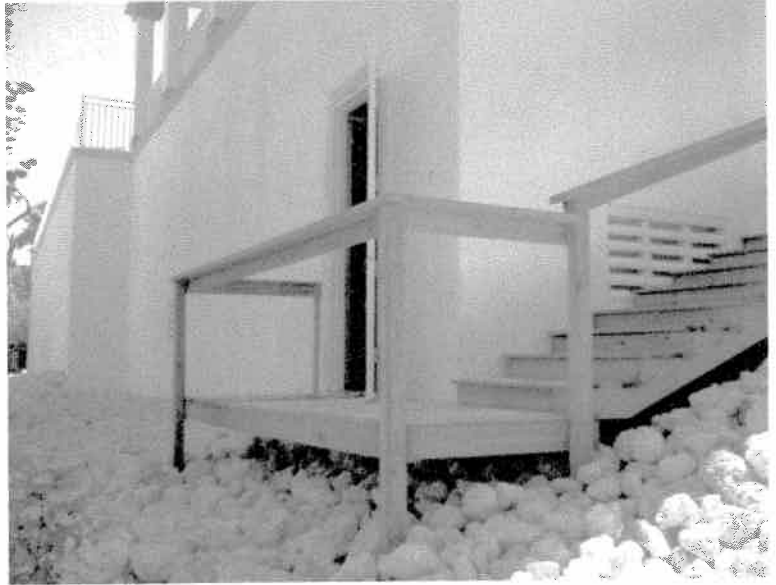
REAR WEST ENCLOSURE DOOR VIEW (04/04/07)
