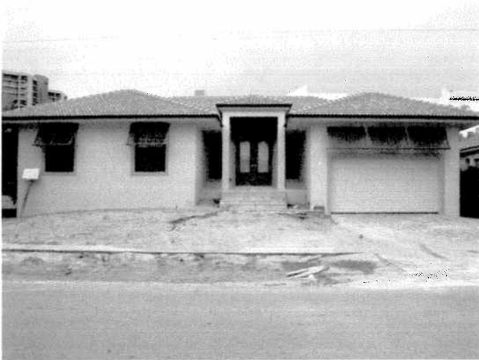
FRONT VIEW (looking West)
