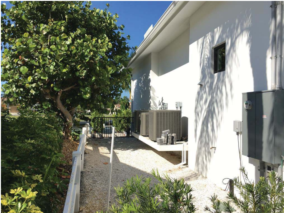
Left Side View from rear of structure 05/17/2019
