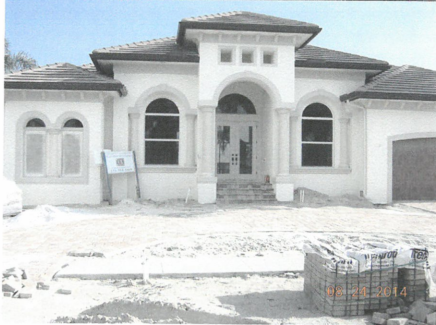
FRONT VIEW (NORTH) August 24, 2014
