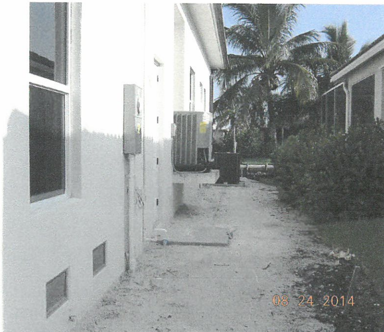
RIGHT SIDE VIEW (WEST) August 24, 2014
