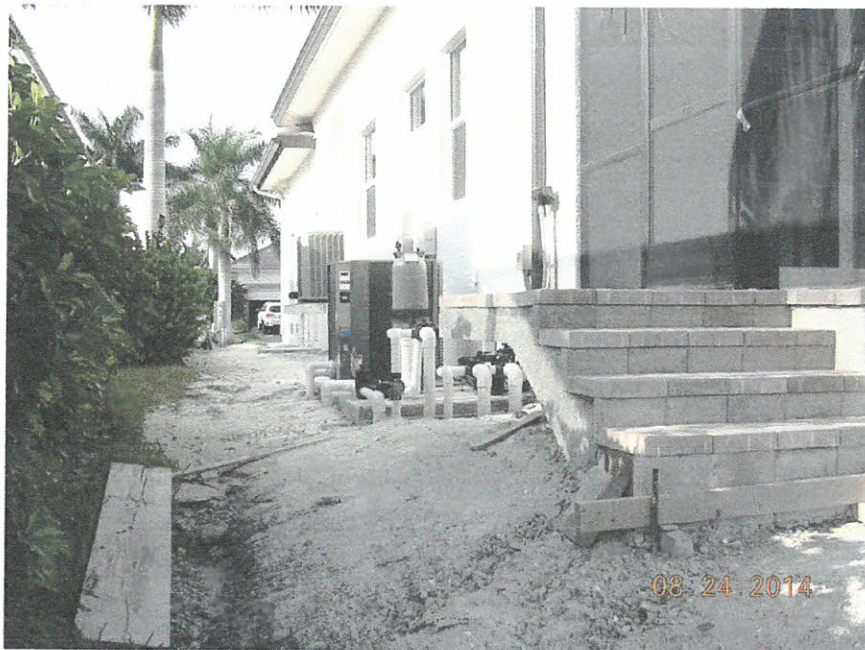
RIGHT SIDE VIEW (WEST) August 24, 2014
