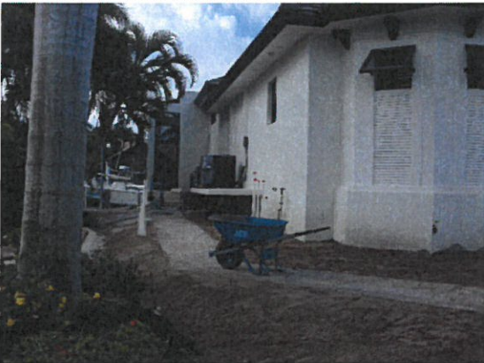
Side and A/C View (East Side)
