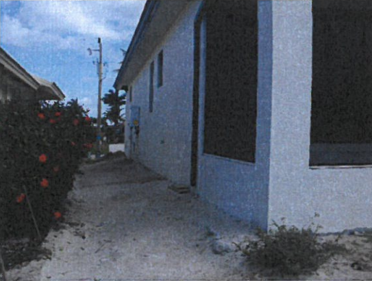
Side View (West Side)
