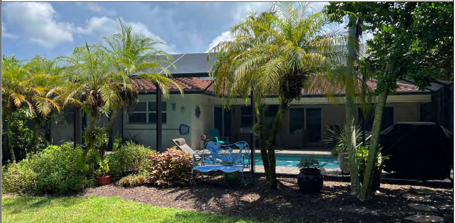
Photo Two Caption REAR VIEW (09/07/2022)
