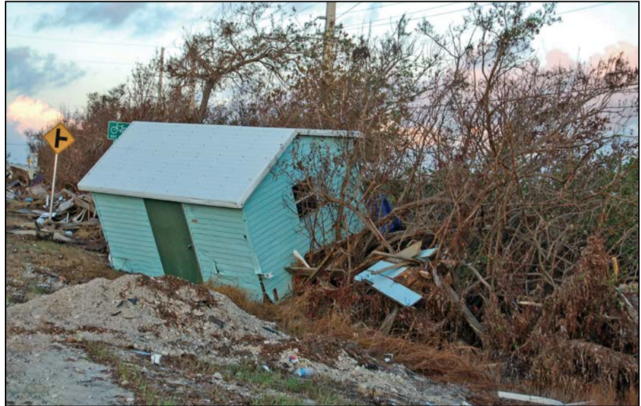
Figure 23: Small accessory structure that was moved by flood and wind forces
