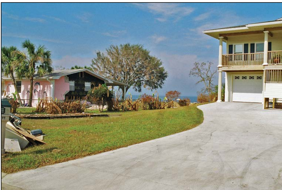
Figure 27: Post-hurricane photo showing an elevated building surrounded by gently sloping fill and an adjacent, damaged, older, non-elevated building
