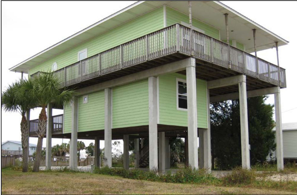
Figure 8: Above-grade enclosure
