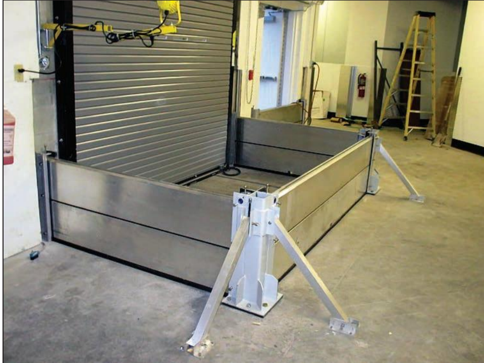
Figure 3: Stop logs deployed inside the building to trap seepage around the garage door and avoid accumulation of rainfall
