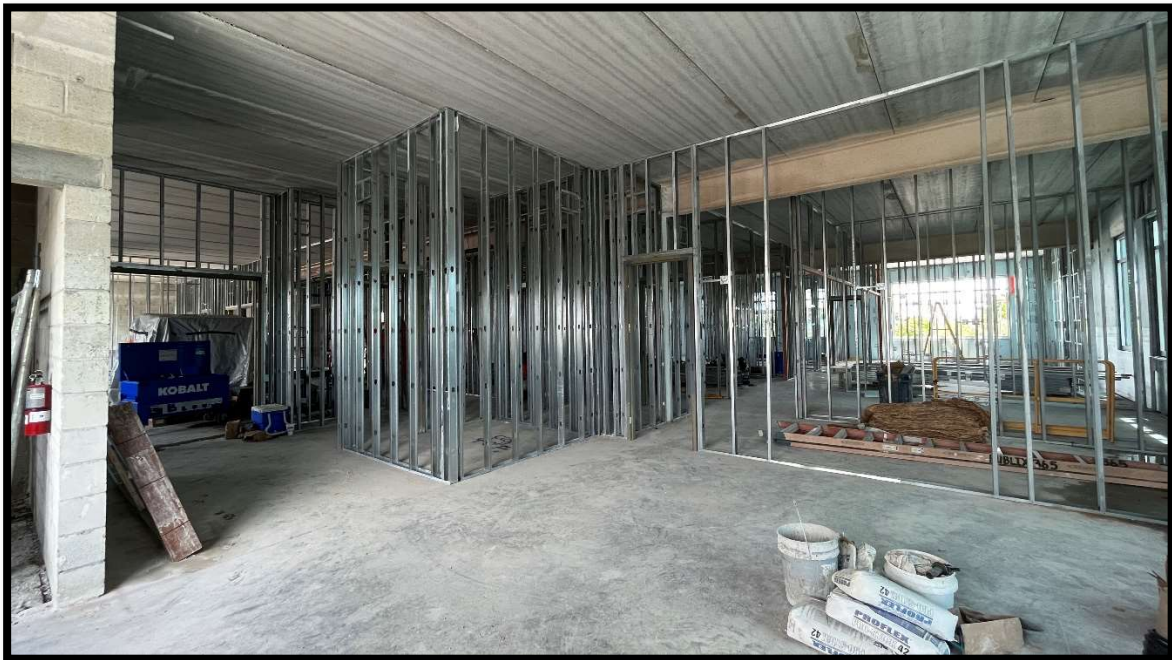
Fire Station 50 – Interior 2 nd Floor Lobby
