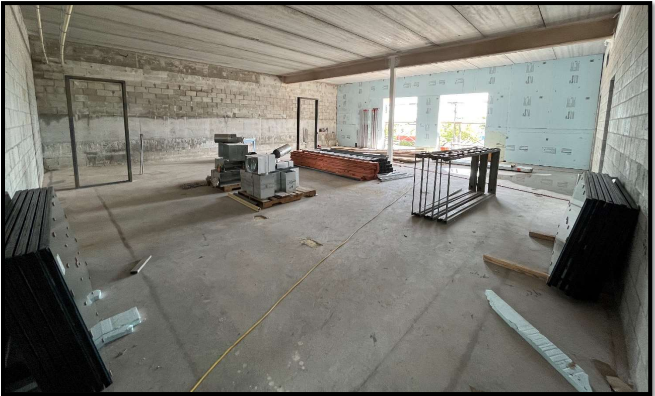
Fire Station 50 – Interior 2 nd Floor EOC
