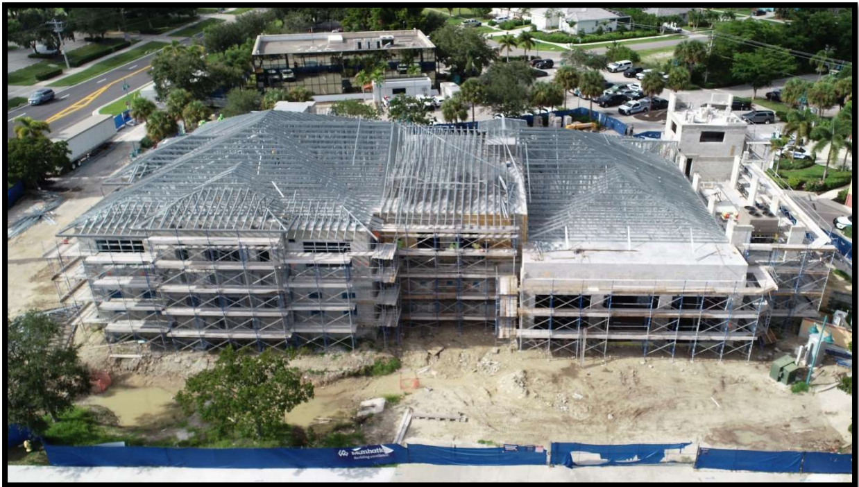
Fire Station 50 – Arial Back of Building
