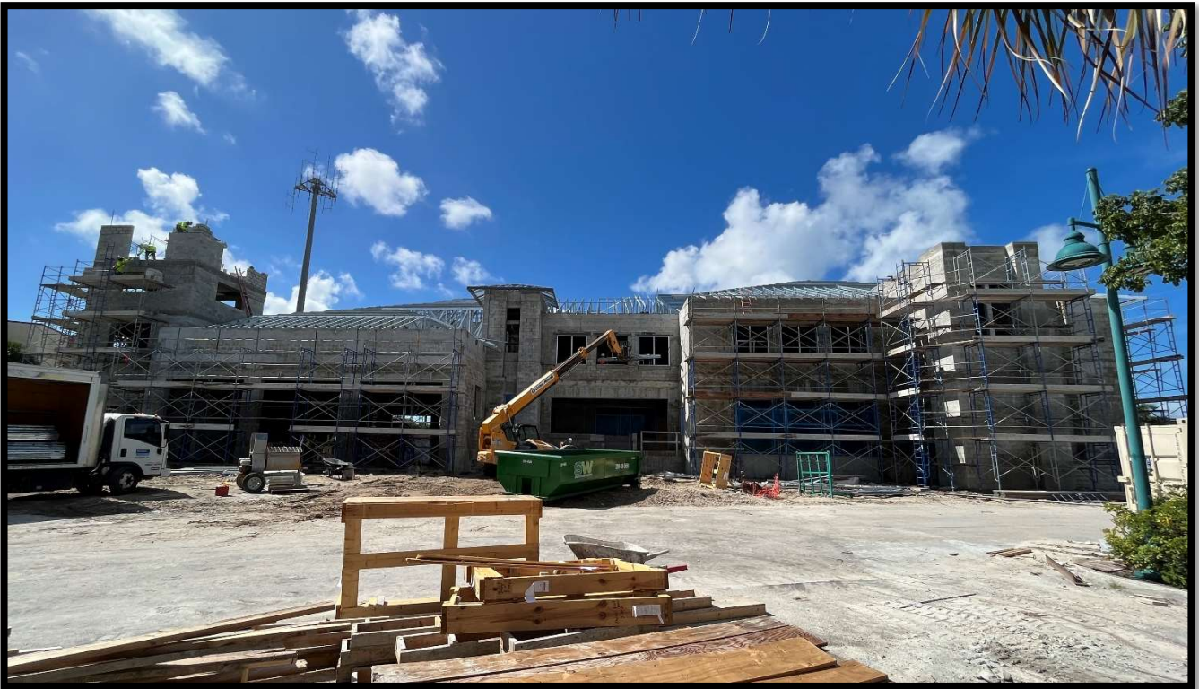
Fire Station 50 – Exterior
