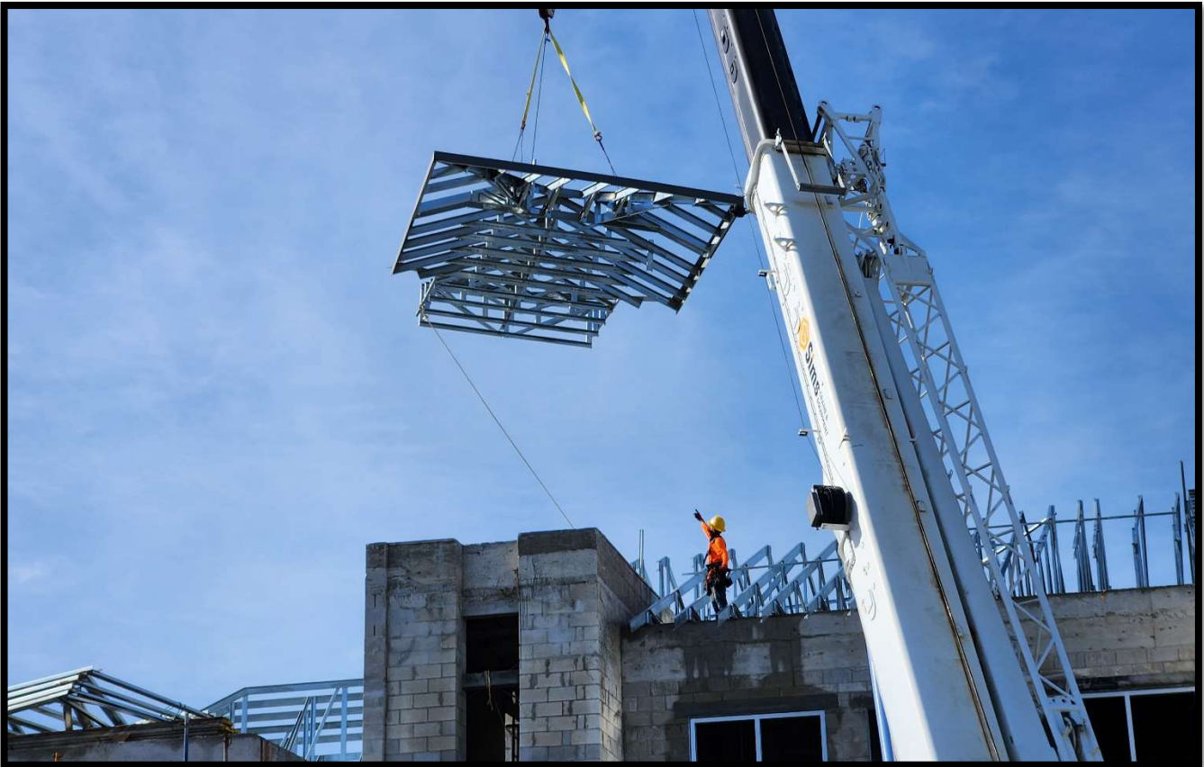
Fire Station 50 – Setting of Roof Trusses
