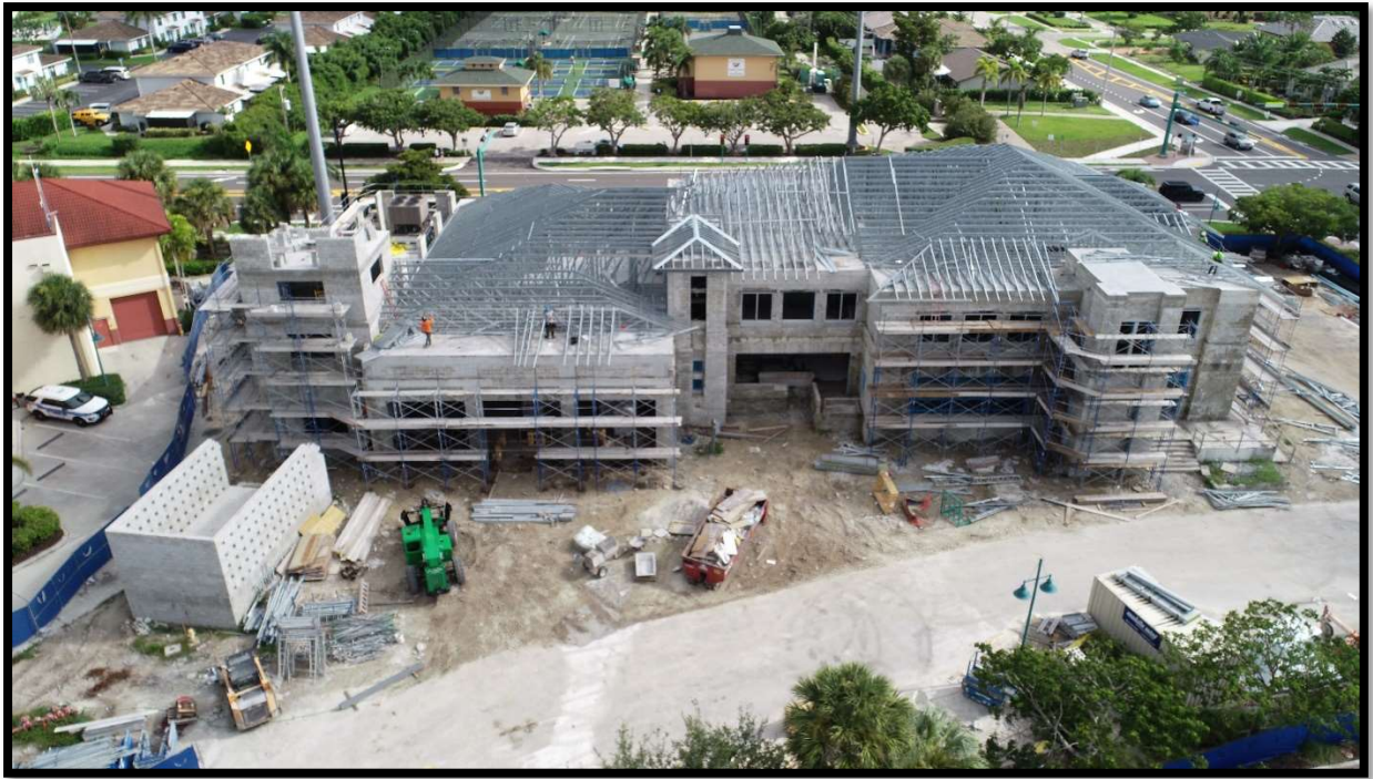
Fire Station 50 – Arial Front of Building
