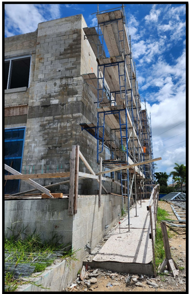
Fire Station 50 – Exterior Block Mitigation in Preparation for Stucco
