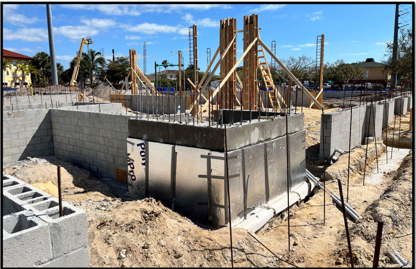
Fire Station 50 – Structure (Elevator Pit)
