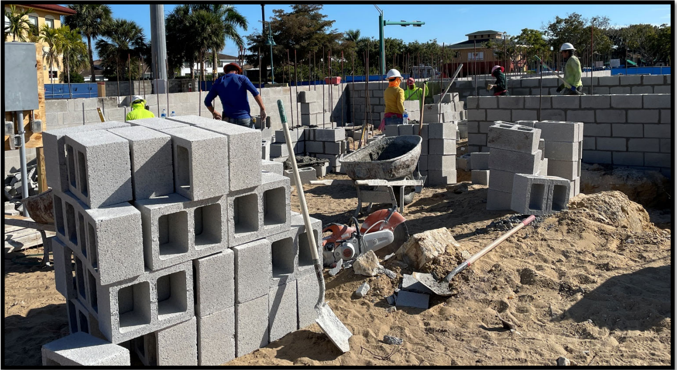
Fire Station 50 – Foundation: Stem Wall
