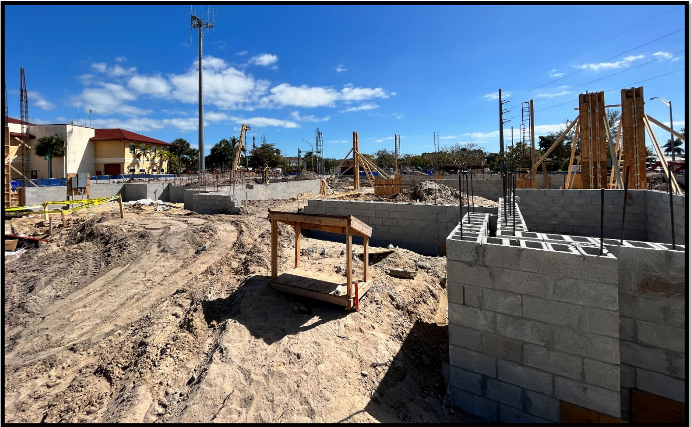
Fire Station 50 – Foundation: Stem Wall & Fill
