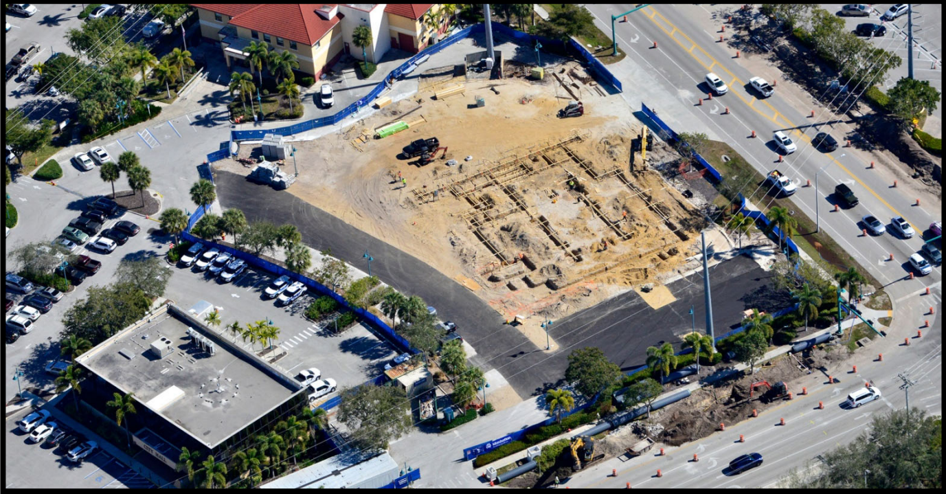
Fire Station 50 – Site Work: Footers
