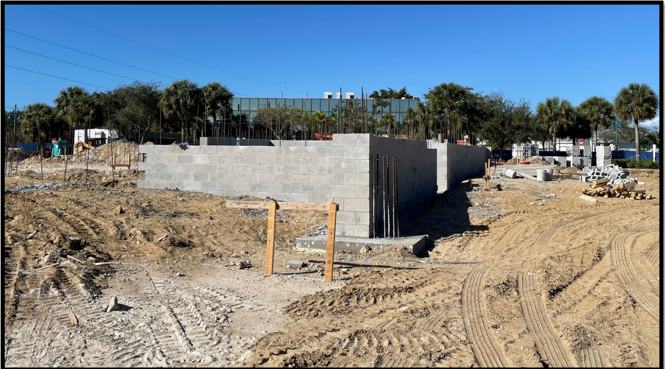
Fire Station 50 – Foundation: Stem Wall
