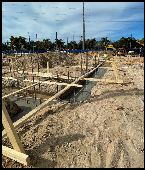
Fire Station 50 – Site Work: Footers
