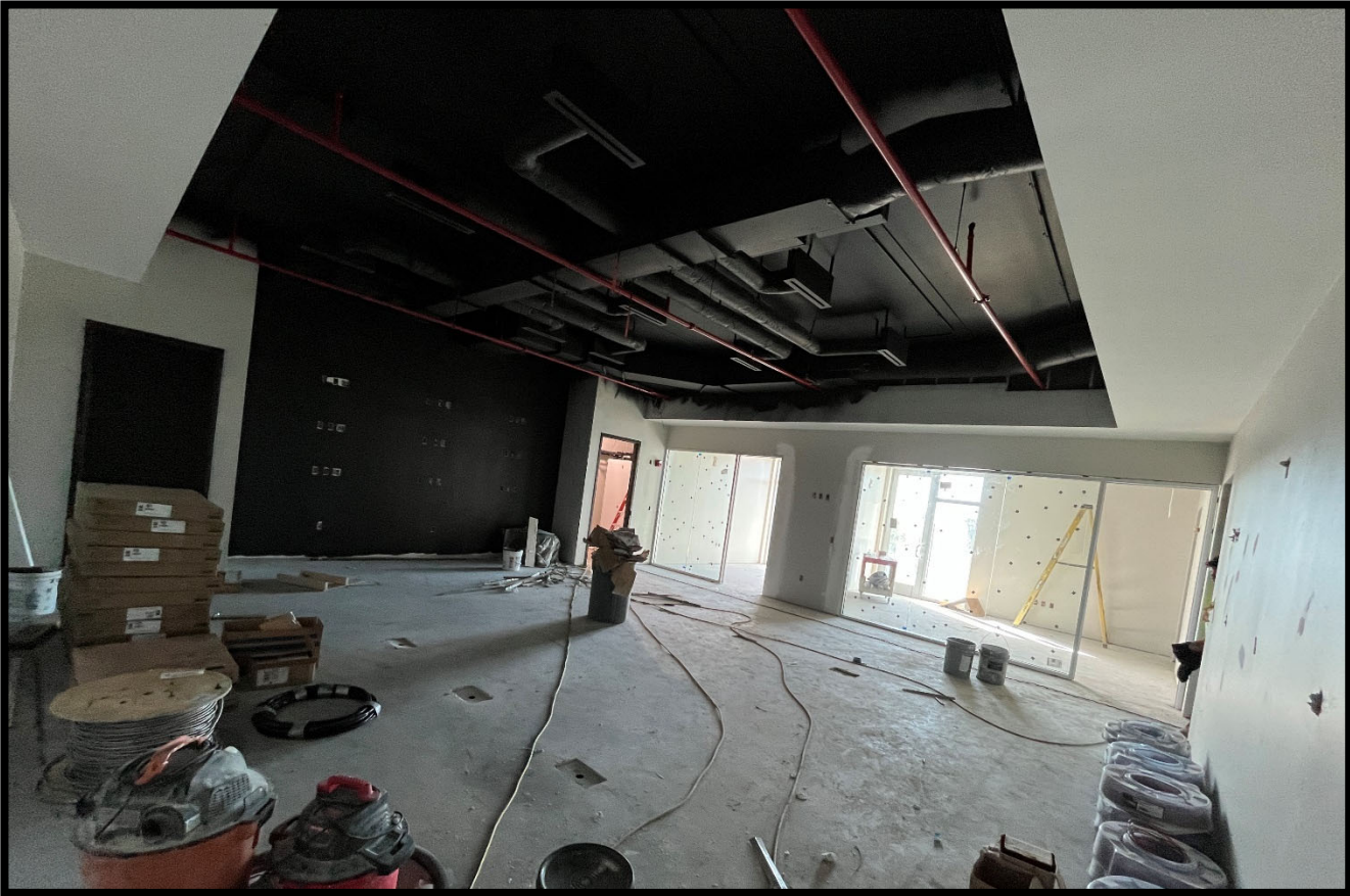
Fire Station 50 – 2 nd Floor EOC
