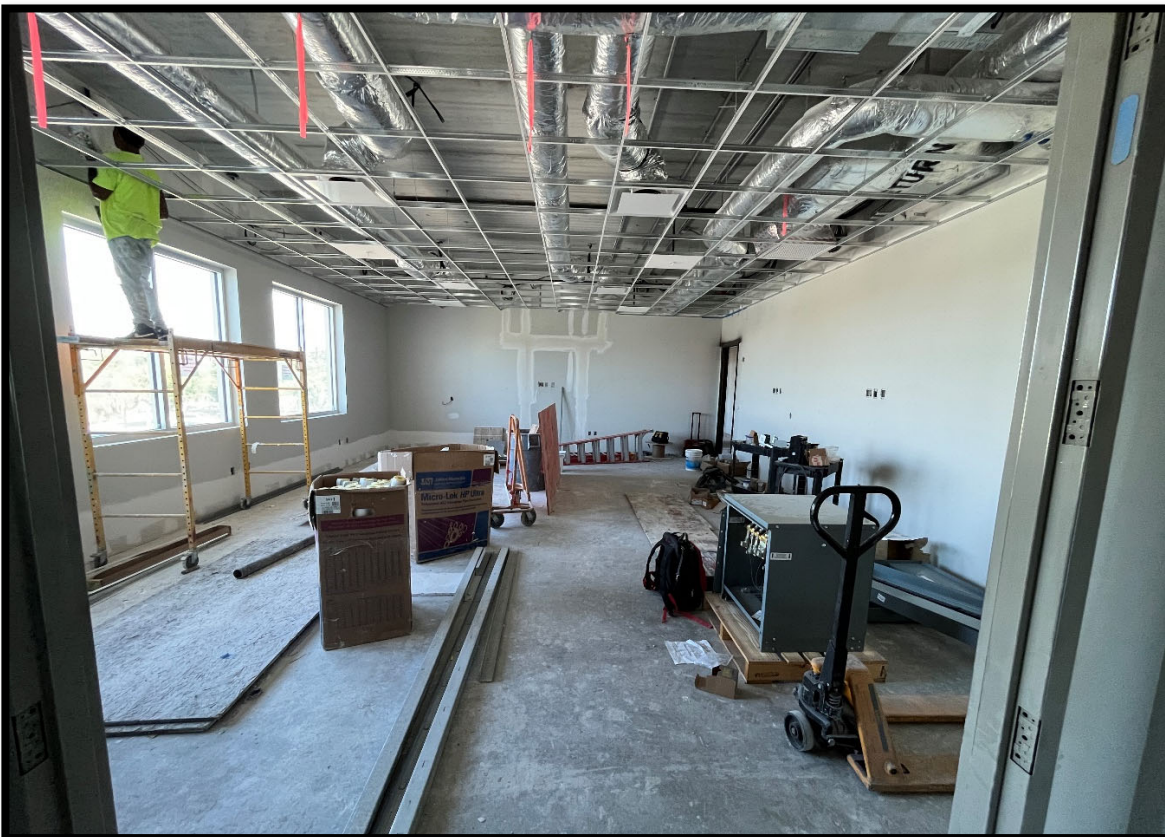
Fire Station 50 – 2 nd Floor Training Room
