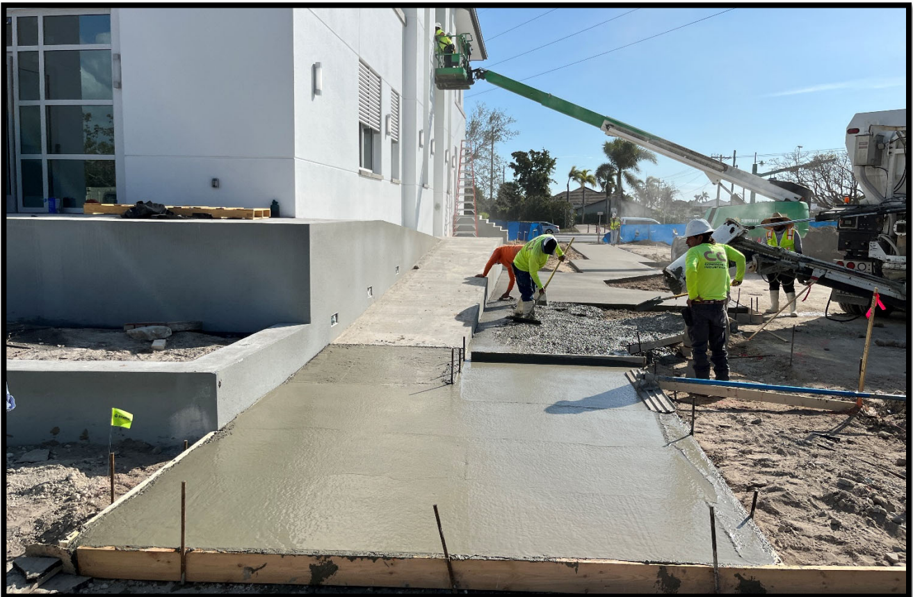
Fire Station 50 – Concrete Work / Sidewalks
