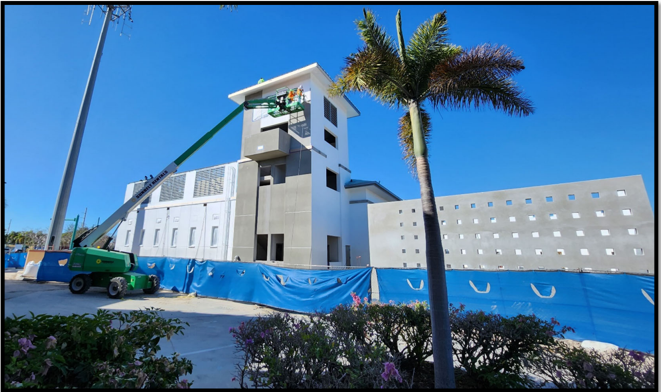
Fire Station 50 – Exterior / Painting
