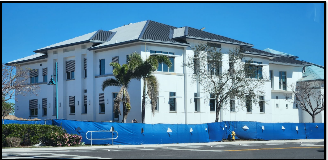
Fire Station 50 – Exterior / Painting
