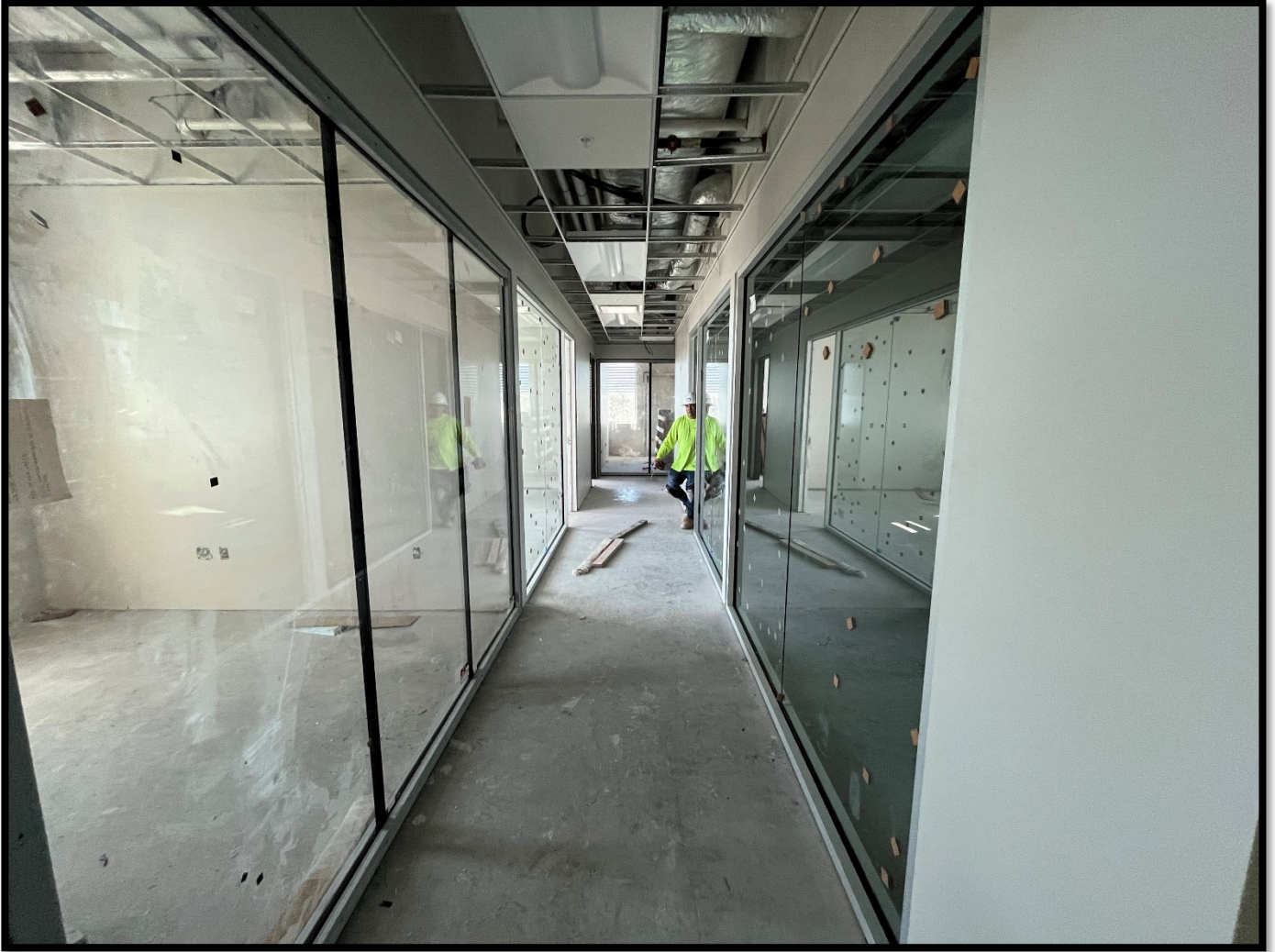
Fire Station 50 – 2 nd Floor Admin Offices
