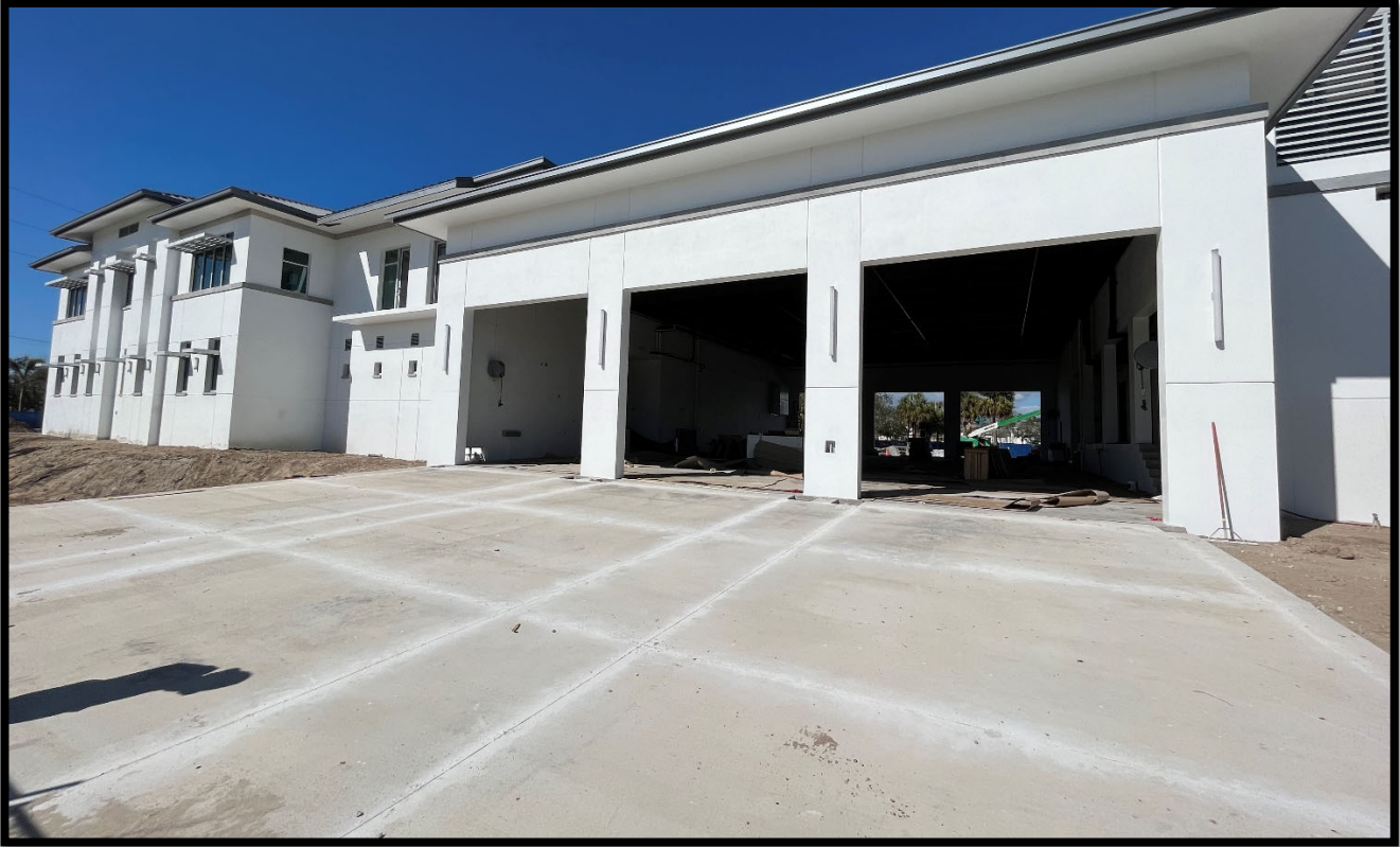
Fire Station 50 – Concrete Apron
