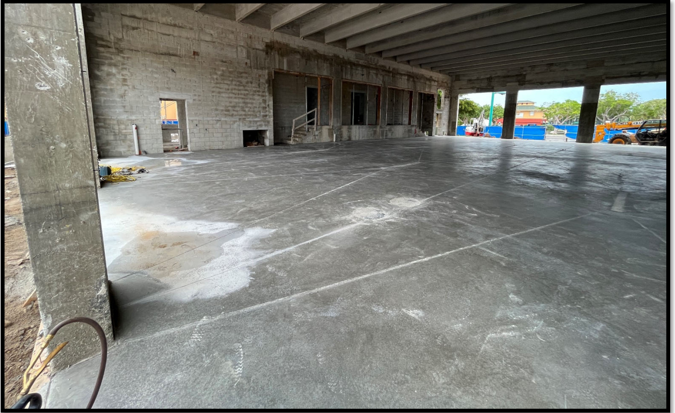
Fire Station 50 – Apparatus Bay Concrete
