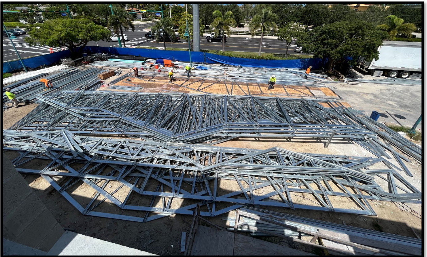
Fire Station 50 – Roof Truss Assembly
