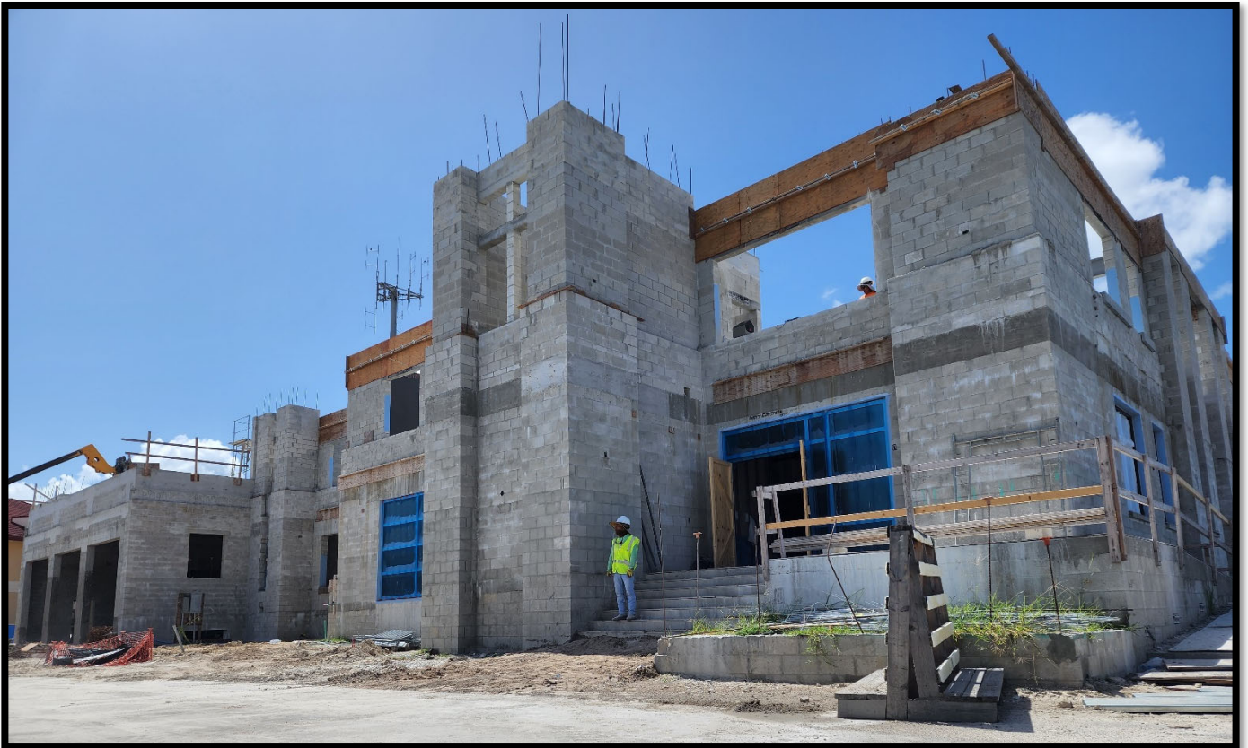
Fire Station 50 – Exterior CMU Block
