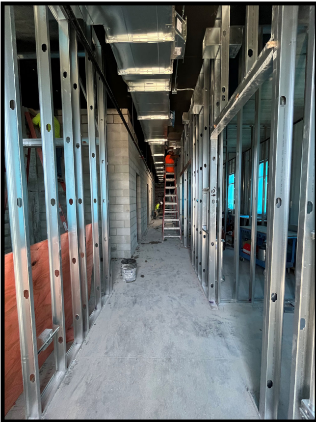
Fire Station 50 – Interior Framing
