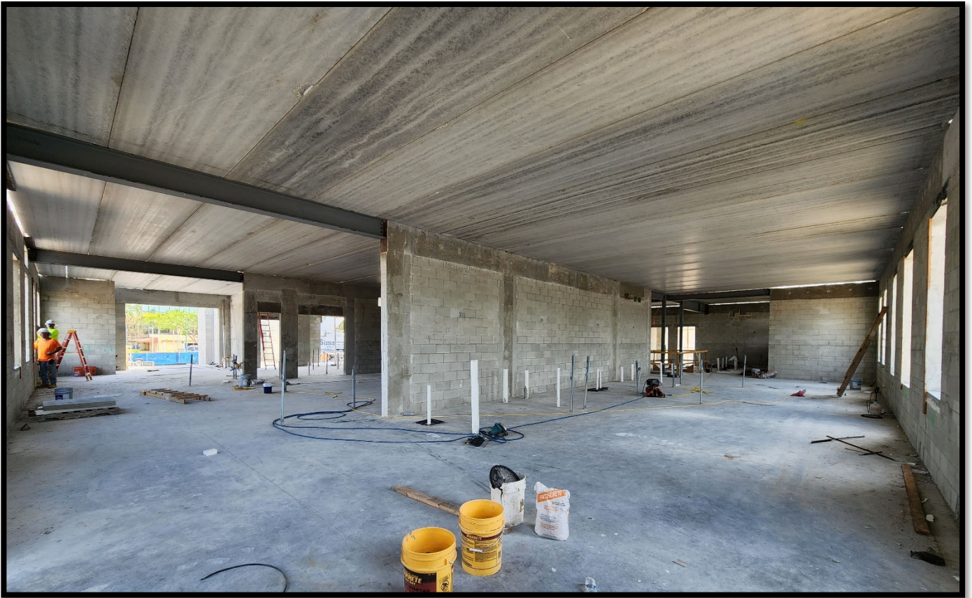
Fire Station 50 – Interior View of Hollow Core Plank
