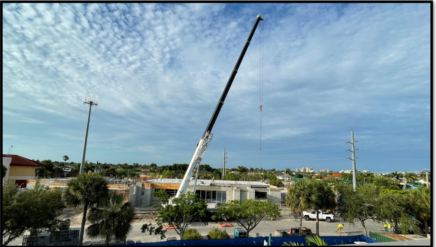
Fire Station 50 – Hollow Core Plank Installation
