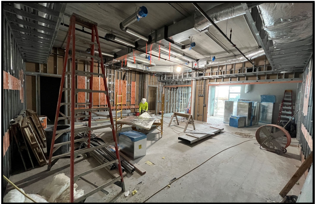
Fire Station 50 – Interior 2 nd Floor EOC
