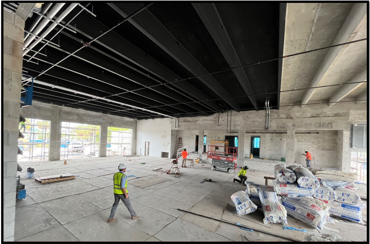
Fire Station 50 – Apparatus Bay
