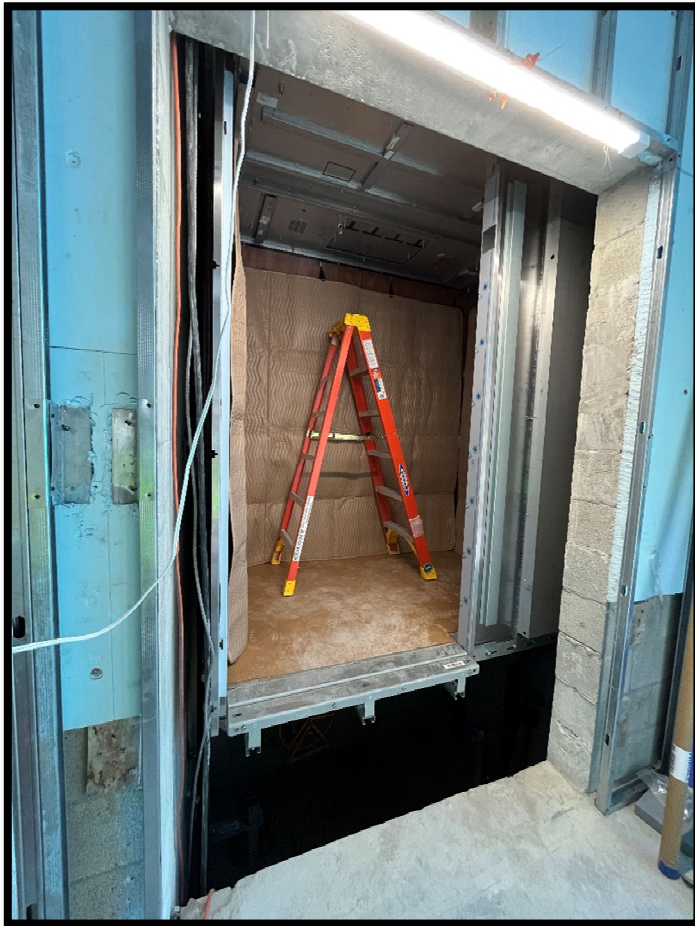
Fire Station 50 – Elevator Installation
