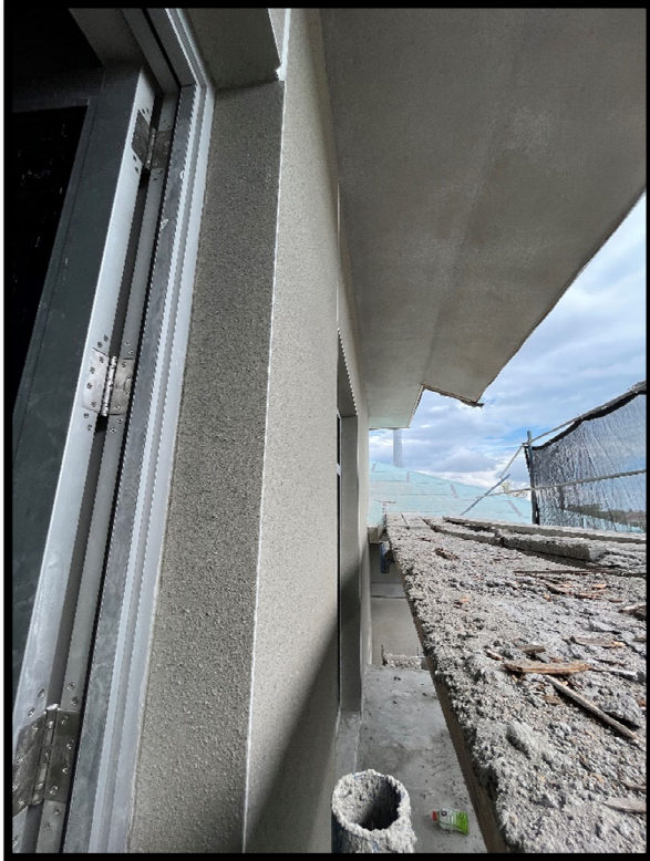
Fire Station 50 – Stucco Installation
