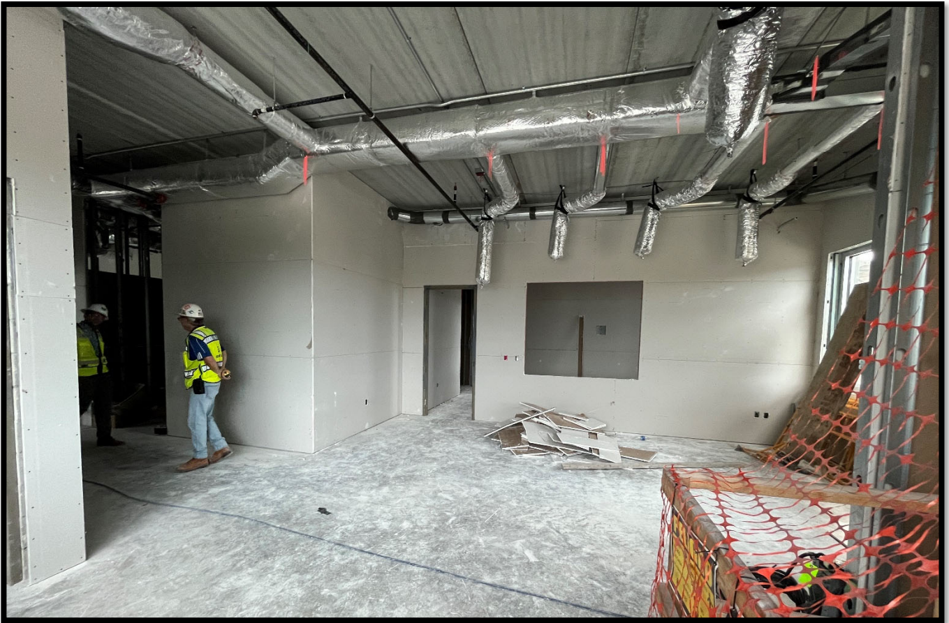
Fire Station 50 – Interior 2 nd Floor Lobby
