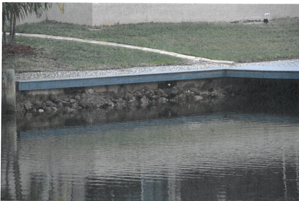
Figure 26: Older seawall with rip rap showing substantial benthic growth
