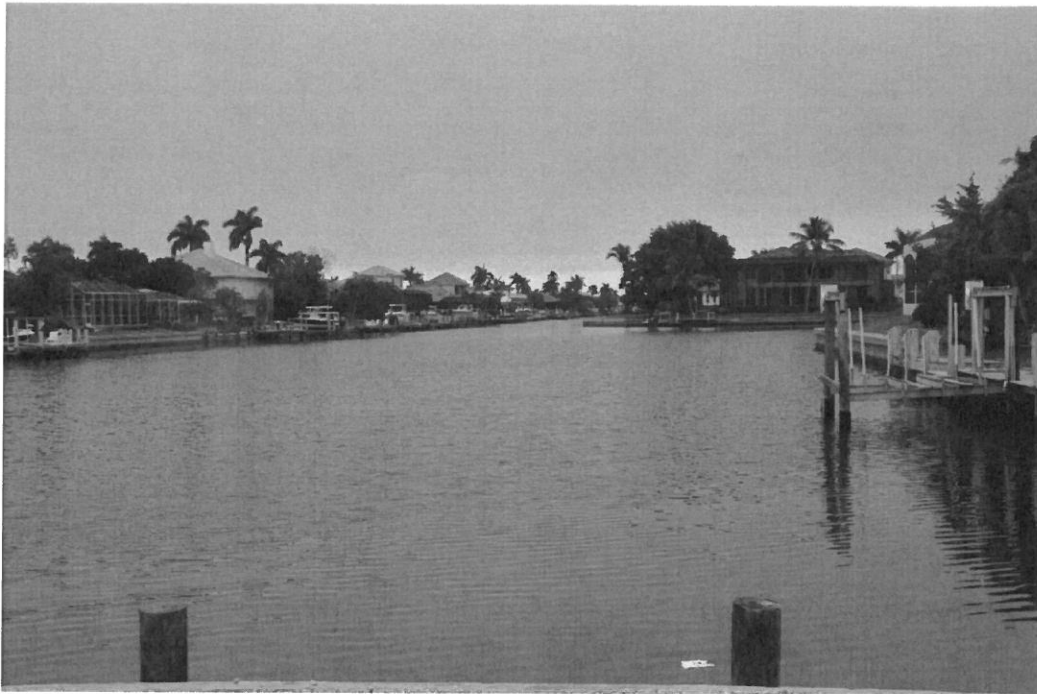
Figure 25: Canal ringed with vertical seawalls
