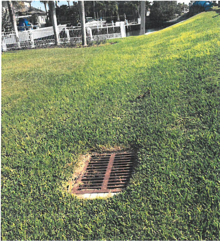
Figure 18: Stormwater grate at the low point of the swale.
