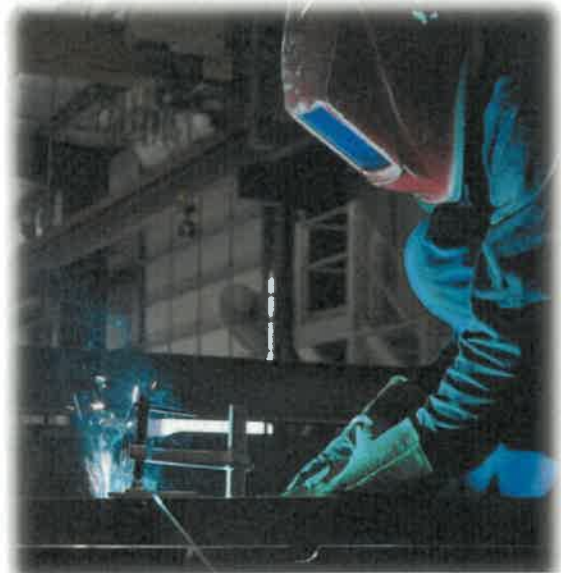
Production Welding in Jeanerette, LA
