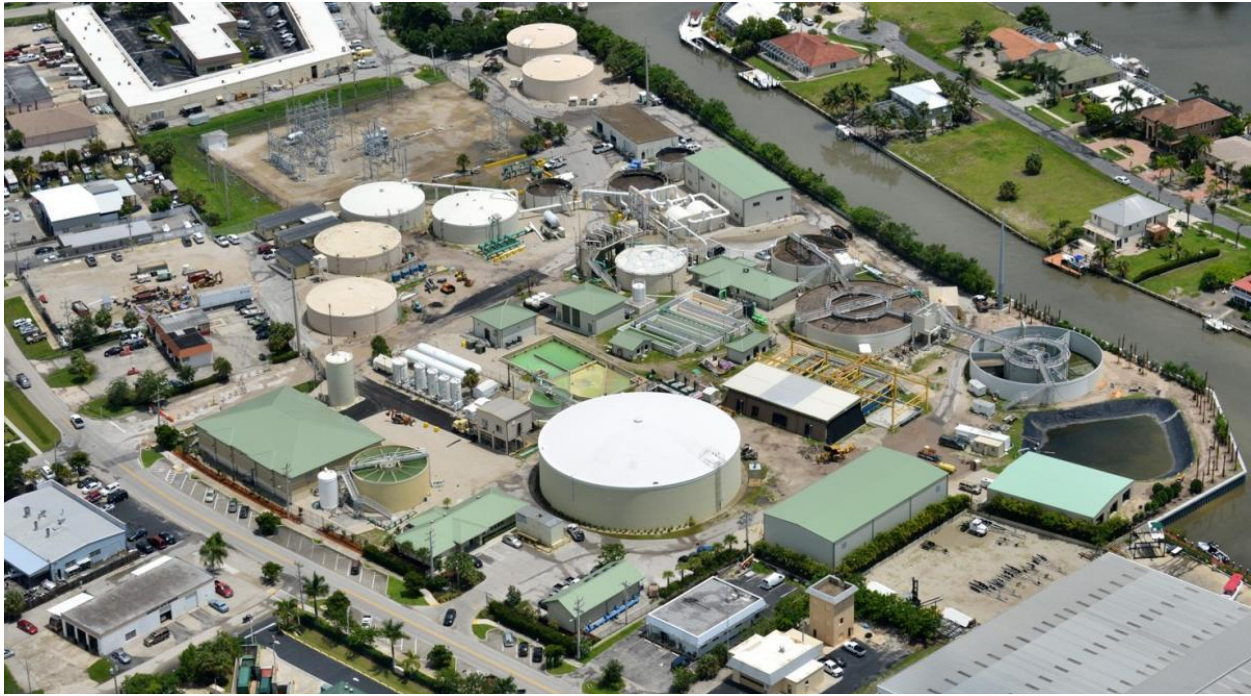
Figure 3-8. Photo of the City of Marco Island Wastewater Treatment Facility. (Source: City of Marco Island)
