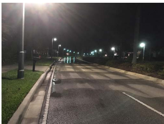
b. Overspray of reuse irrigation along Collier Blvd.
