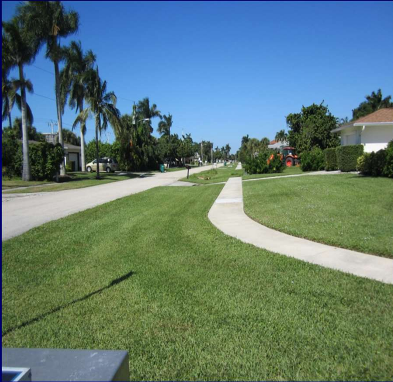
Swale system between storm events
