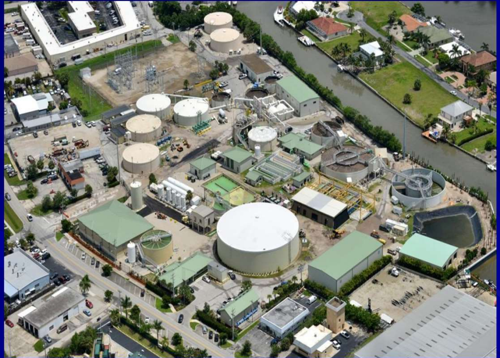
Marco Island Reclaimed Water Production Facility
