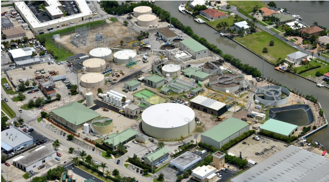
Figure 3-8. Photo of the City of Marco Island Wastewater Treatment Facility. (Source: City of Marco Island)
