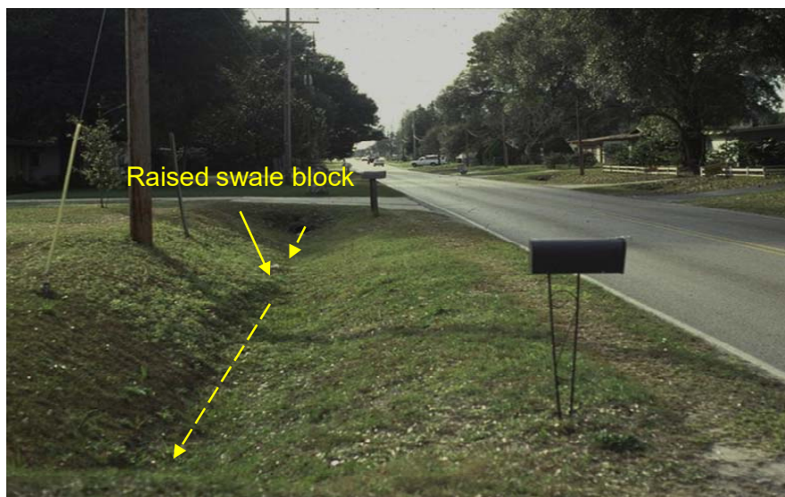
Figure 7-3. Example of a Typical Swale Block.
