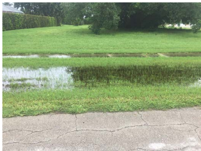
b. Swale system during storm events
