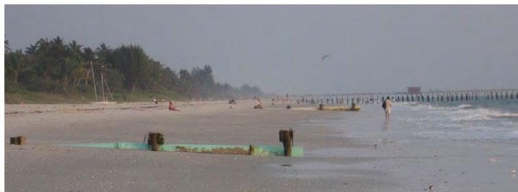
Figure 1-3. Typical Outfall Blockage (Outfall 9)
